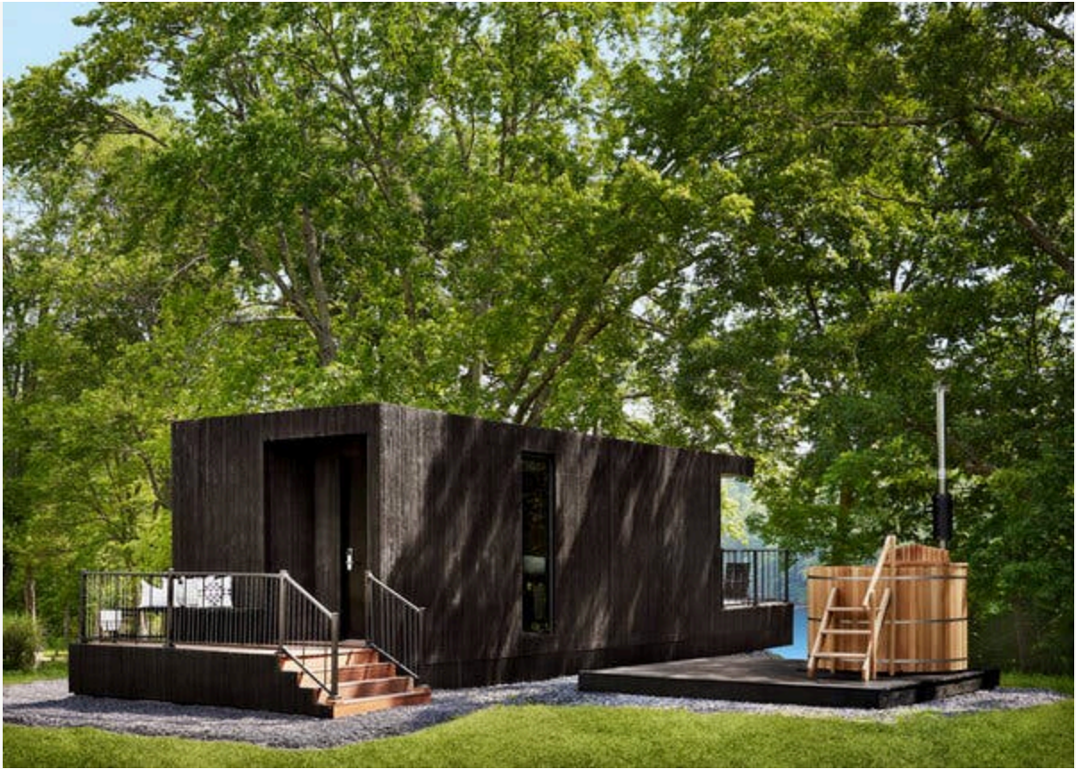
Each Moliving unit is mobile, set on permanent wheels disguised by skirting after installation.Credit...David Mitchell
